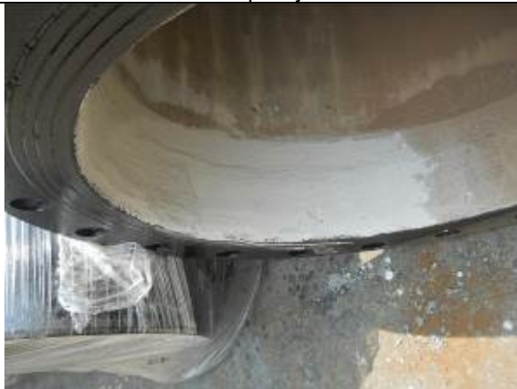
Repaired by manufacturer
