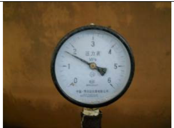
Hydraulic pressure test
