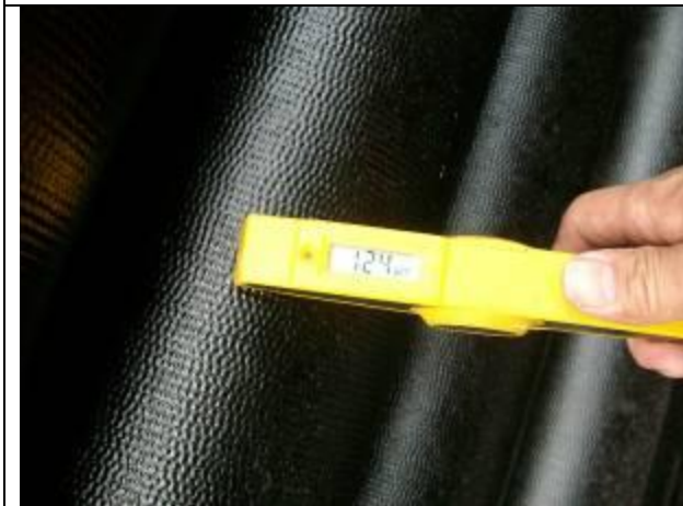
Bitumen coating checking
