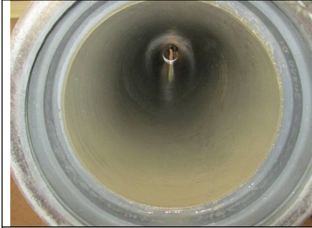
Pipe after lining
