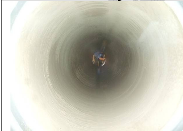
Cement lining check and repair
