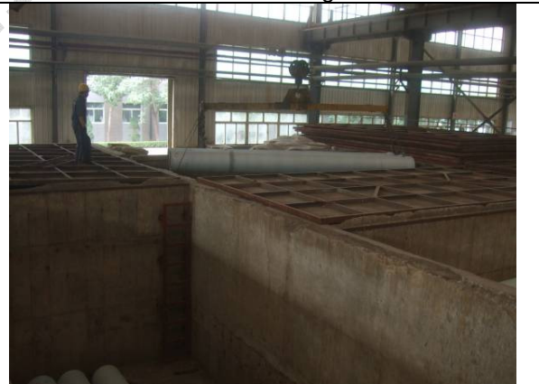
Cement lining preserve
