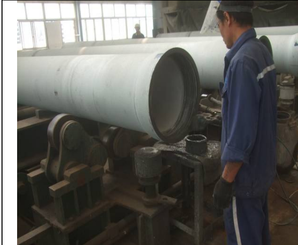
Coating the socket use the zinc rich paint
