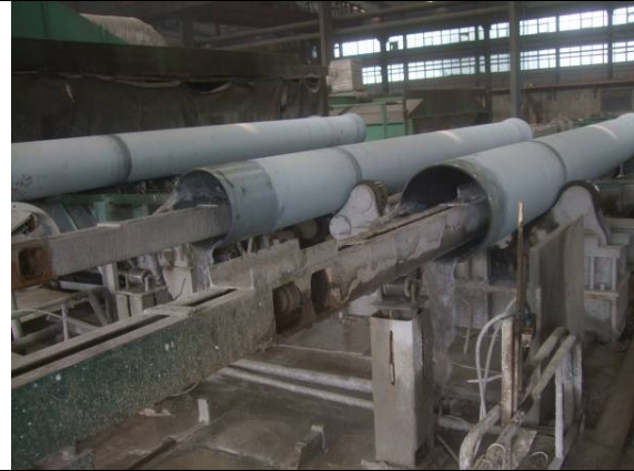
Polish the cement lining
