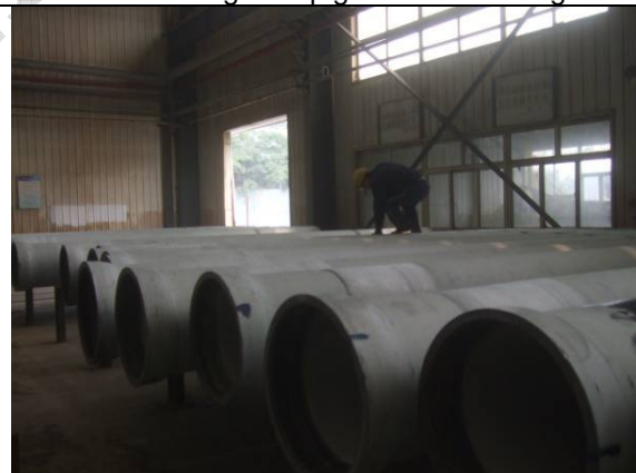
Visual inspection before coating
