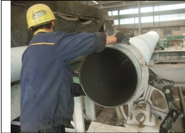
Spigot re-check before coating
