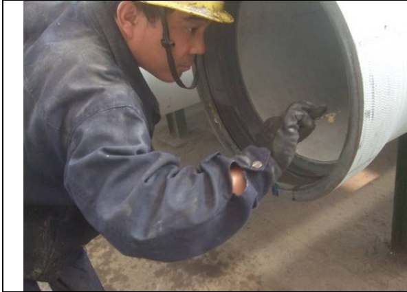
Socket check and slag pocket repair
