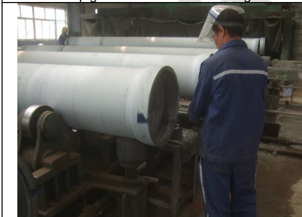
Re-Grinding the socket before coating
