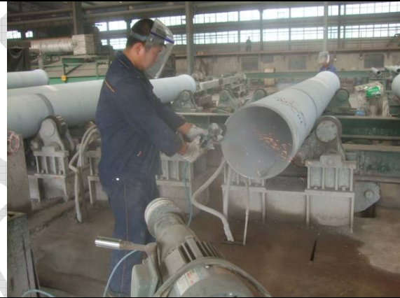
Re-Grinding the spigot before coating
